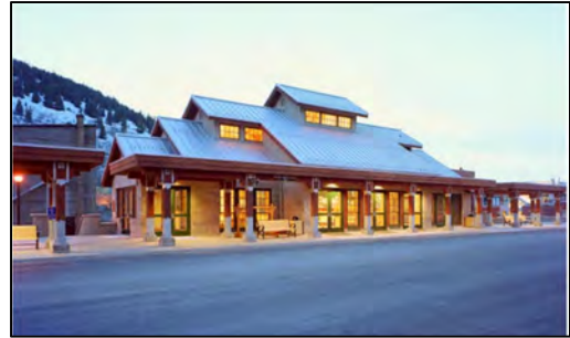
Figure B-25 Park City Transit Center
